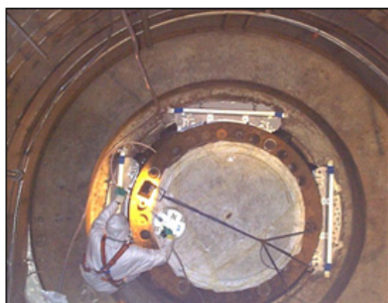
NST Sealing for RPV Dismantling
