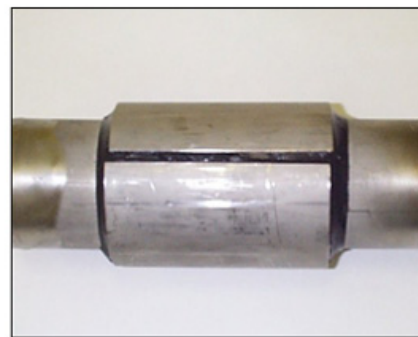
Pipe Repair (retaining clamp)
